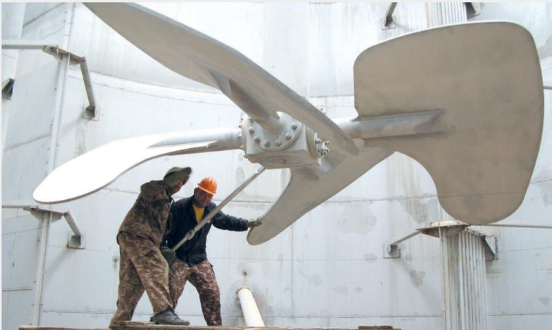
Installation of a large ISOJET B for hydrometallurgy
